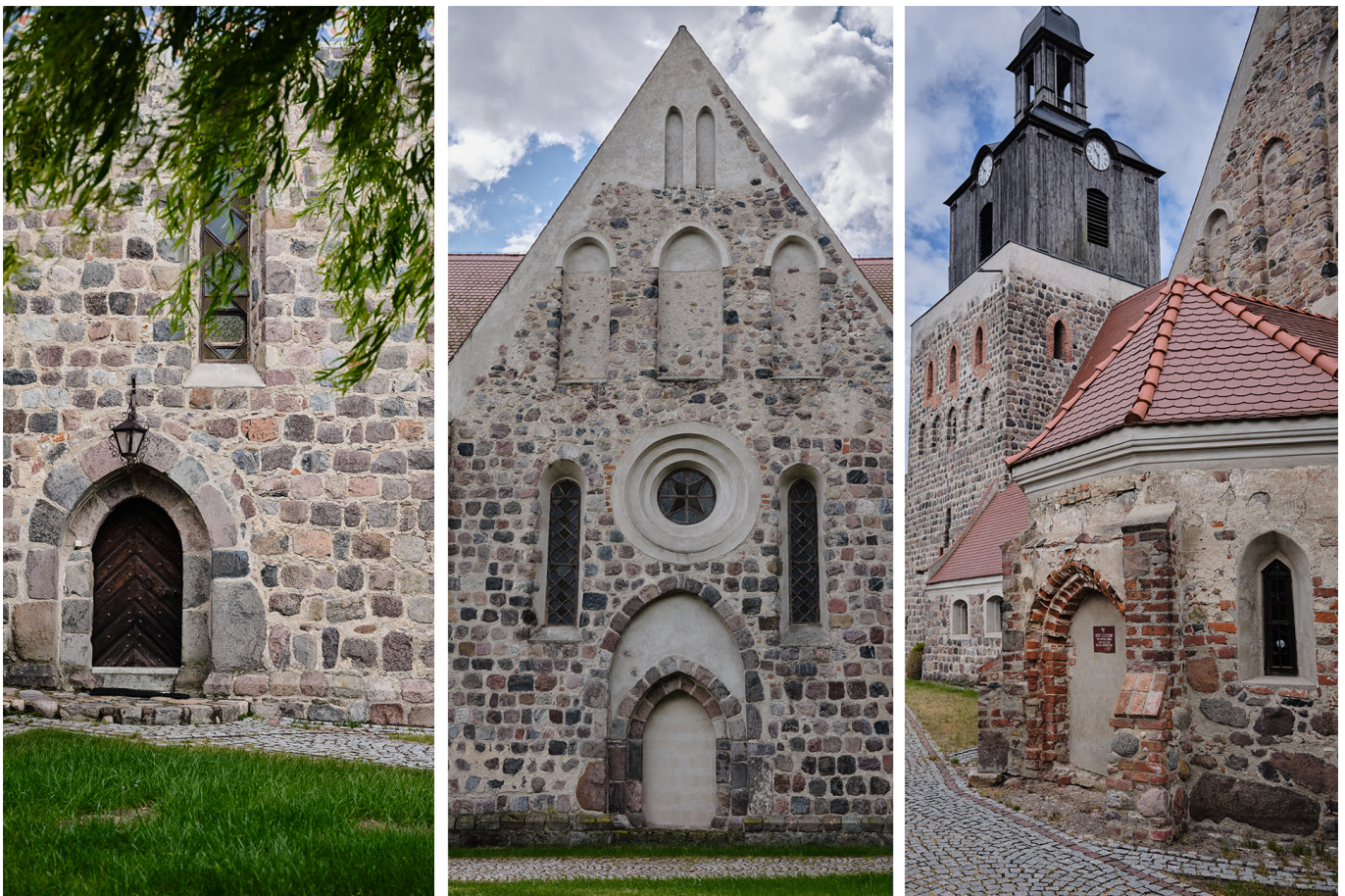
South elevation, north elevation, sacristy / fot. Aleksander Pukalski / Moryń 2025.
